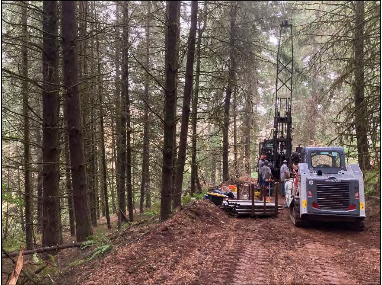
Drilling performed with track-mounted CME rig, operated by Western States Drilling, on February 16 through 18, 2021 and HazTech Drilling on November 8 through 16, 2022. Note the skid steer and cleared road required for site access.
