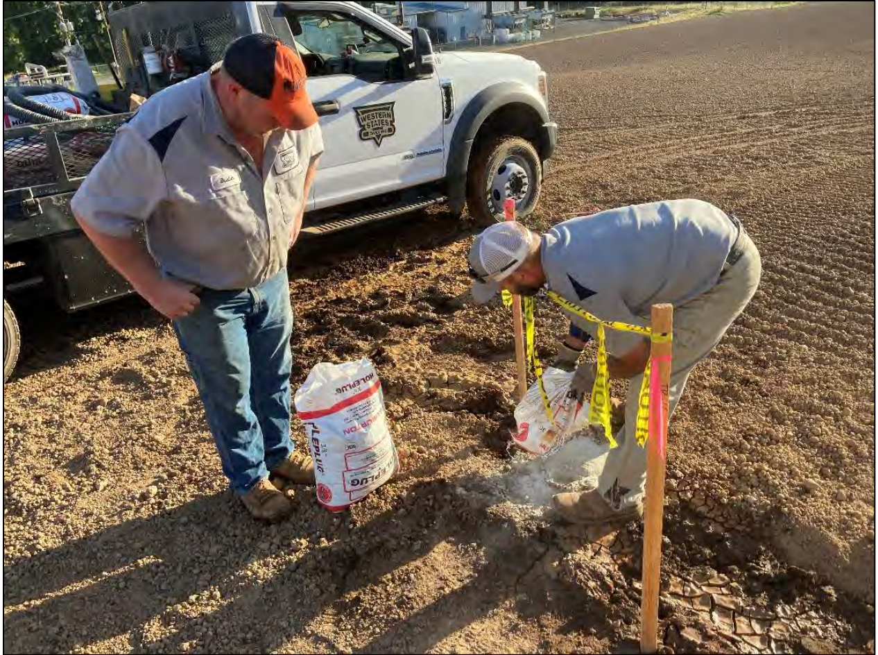
Borings were backfilled using bentonite.
