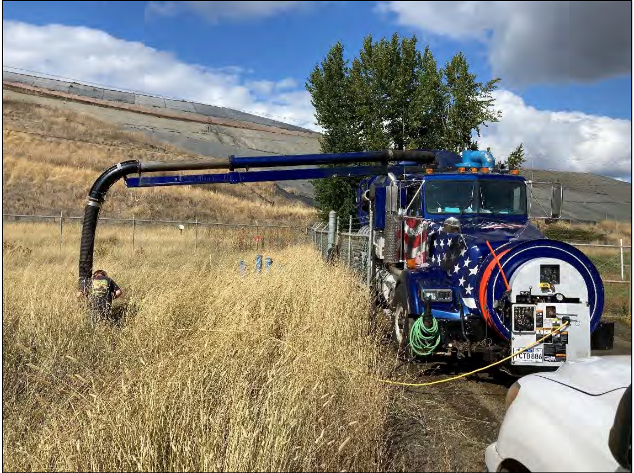
Areas near known landfill utilities were advanced using a vacuum truck.
