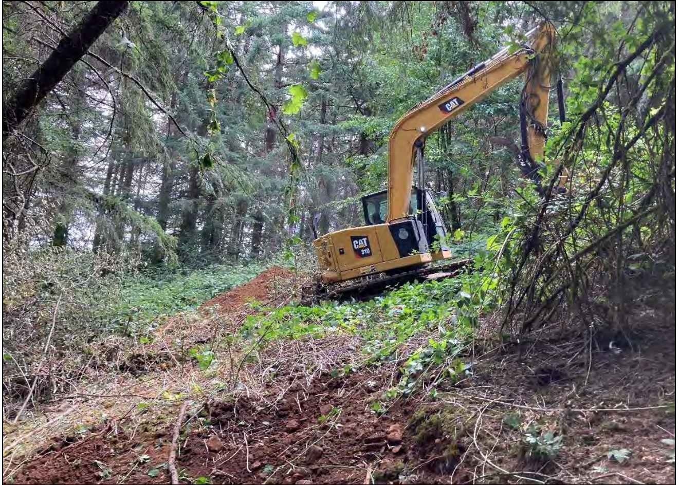
Test pits were located to provide access to the proposed boring locations, and the excavator was used to clear and grade access to the borings.
